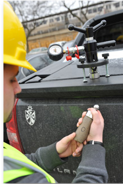
Core Indicating Failure at the Bond Between the Overlay and Substrate
